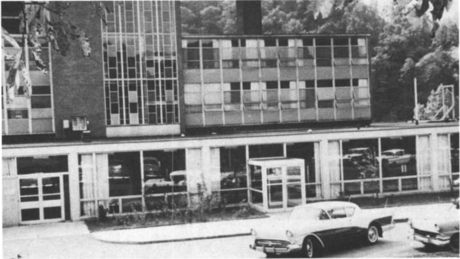
Original Hospital at Hazard
