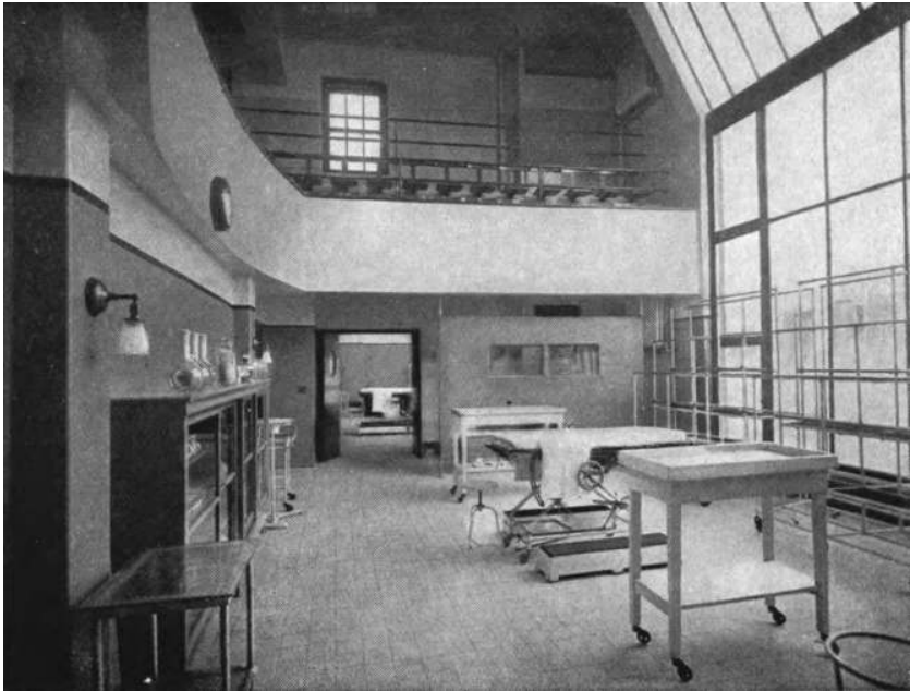
Figure 7. The operating room at Peter Brent Brigham hospital features a full wall of canted glass that served to illuminate the patient during surgery. Published in Peter Bent Brigham Hospital (Boston: Barta Press, 1915?).
